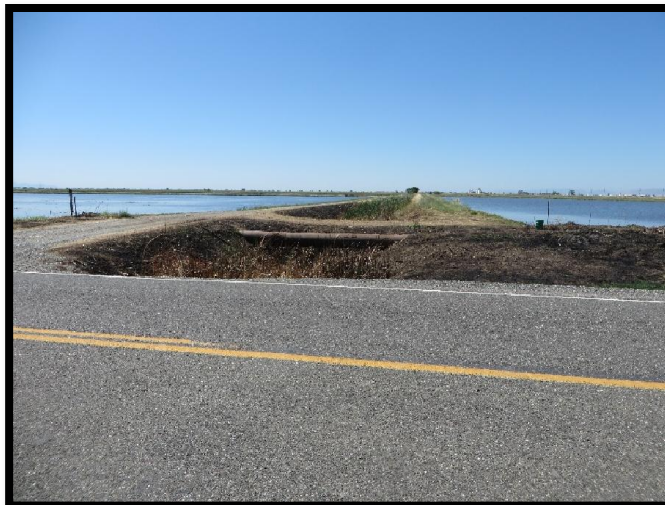
View facing north from County Road 57
