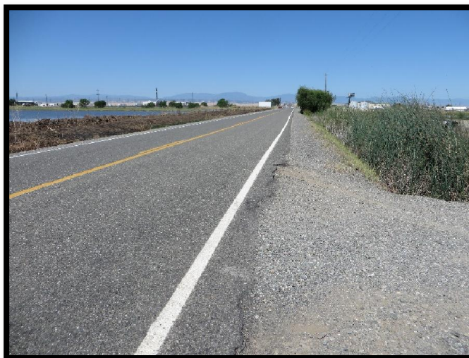
View facing west on County Road 57 from proposed Parcel 1
